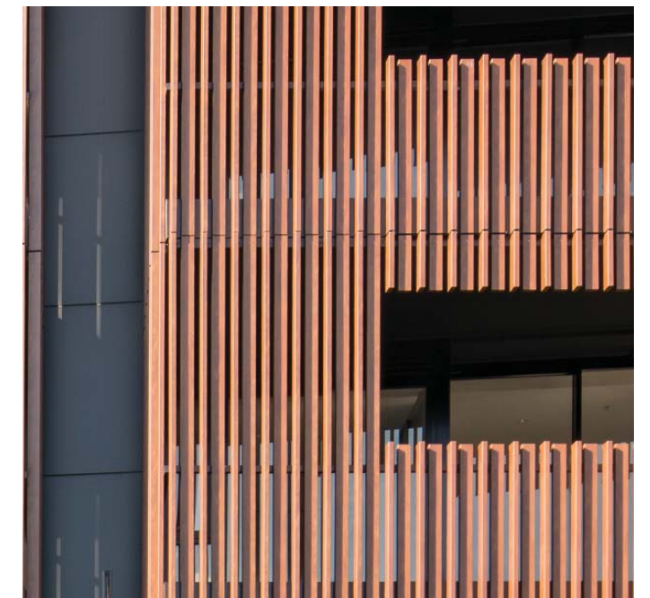
TIM01 - ALUMINIUM SCREENING BATTENS SYSTEM WITH WOOD GRAIN FINISH - KNOTWOOD SPOTTED GUM OR SIMILAR
