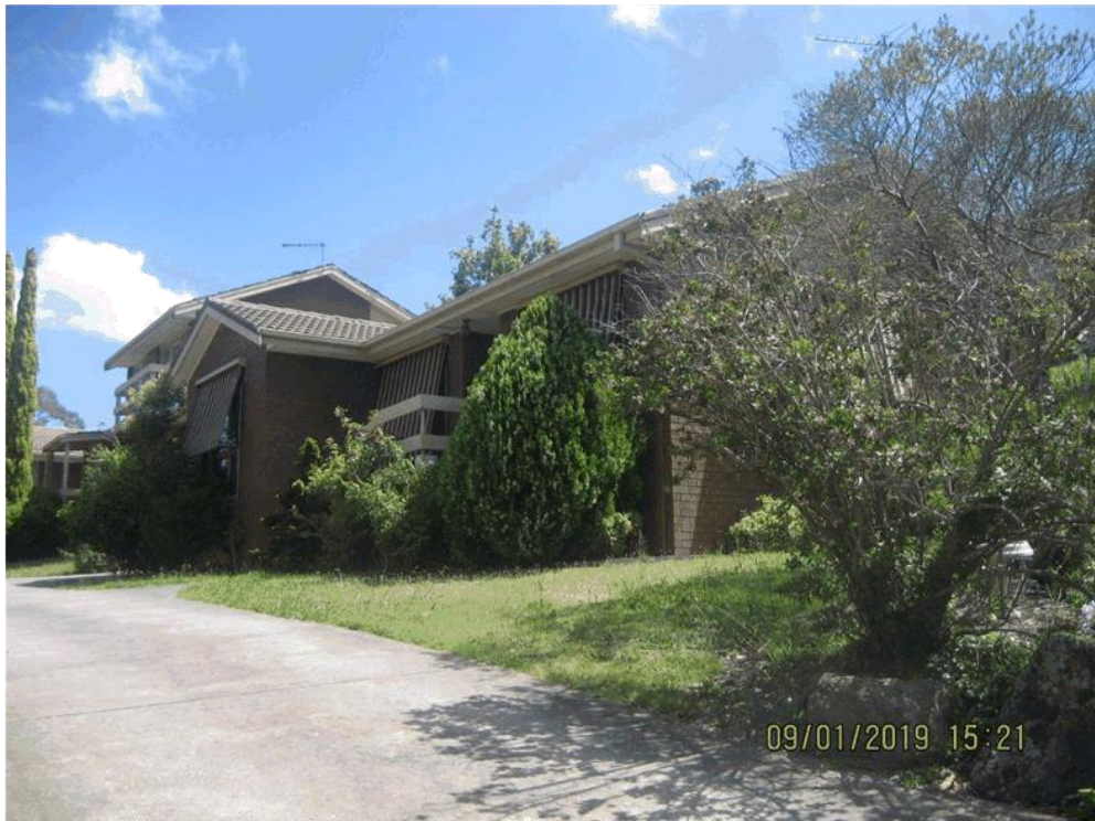
Multi-unit development at 18-20 Glendale Avenue, immediately opposite subject land.
