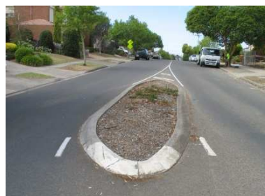
Poor Garden Bed – Grant Olsen Ave - Manningham
