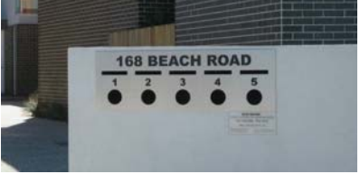
No. 4 Letter Box Brick Structure With Render
