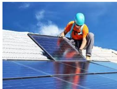
Solar panel installation
