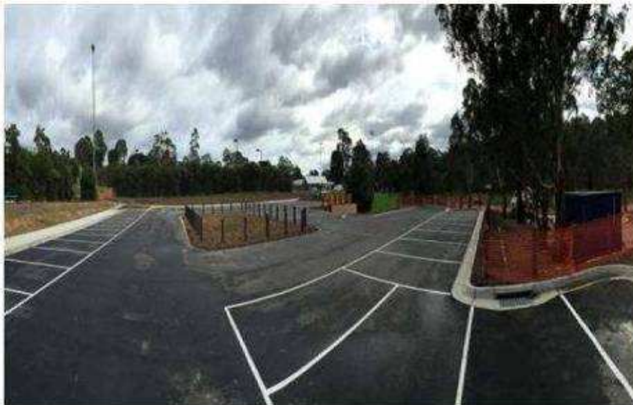
Mullum Mullum Highball Facility - Car Park and Early Works
