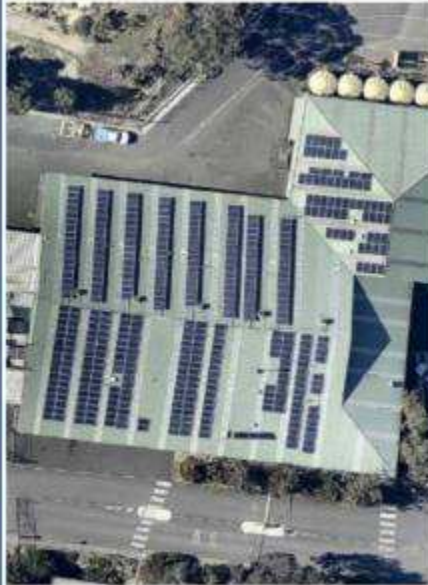
Depot rooftop with completed 99kW Solar PV array
