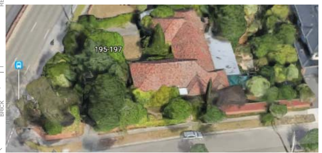
AERIAL VIEW FROM ROSEBANK TERRACE
