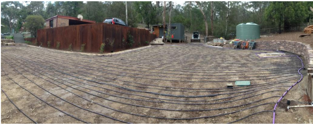
Figure 5: Lay-down of sub-surface irrigation
