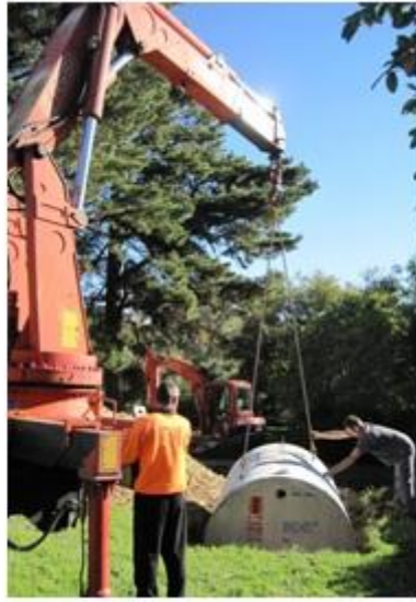
Figure 4: Septic system components in various stage of construction/installation
