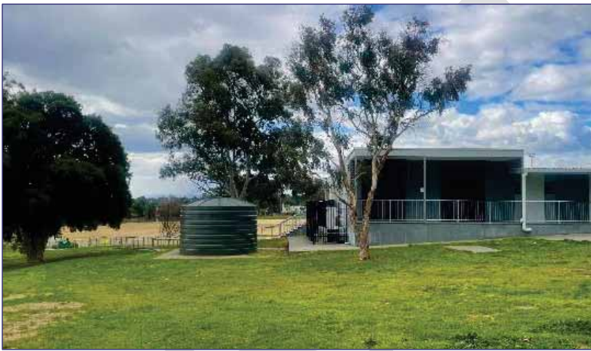
Figure 6: Rainwater tank at Schramms Reserve, Doncaster used for toilet flushing. An additional rainwater tank is located underground to water the sports oval
