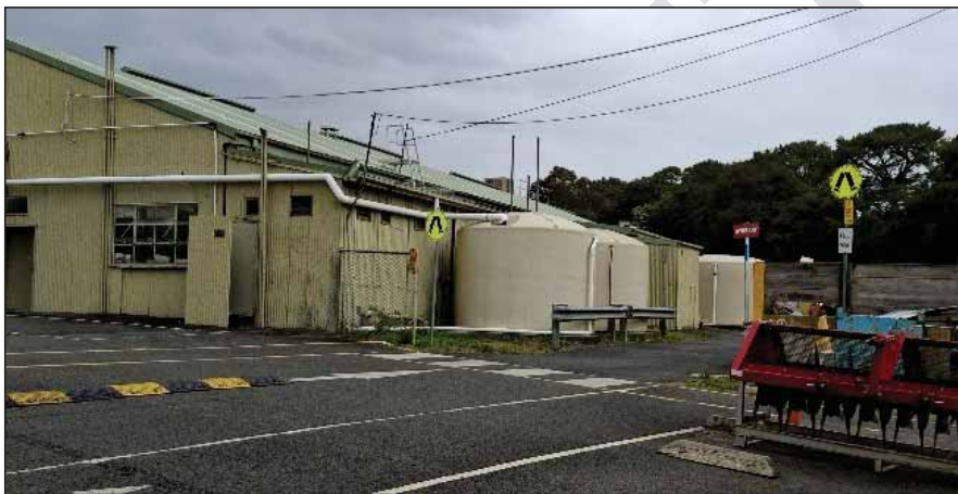
Figure 7: Rainwater Tanks at the Manningham Council Depot Site, Doncaster East
