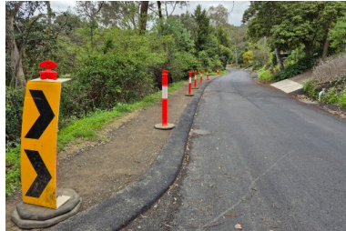
Melbourne Hill Road Drainage
