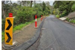
Melbourne Hill Road Drainage
