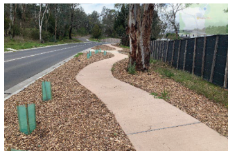
Jumping Creek Road
