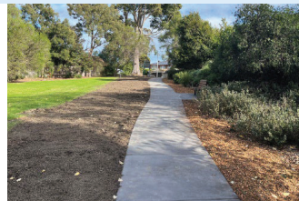
Tolsoy Footpath Construction
