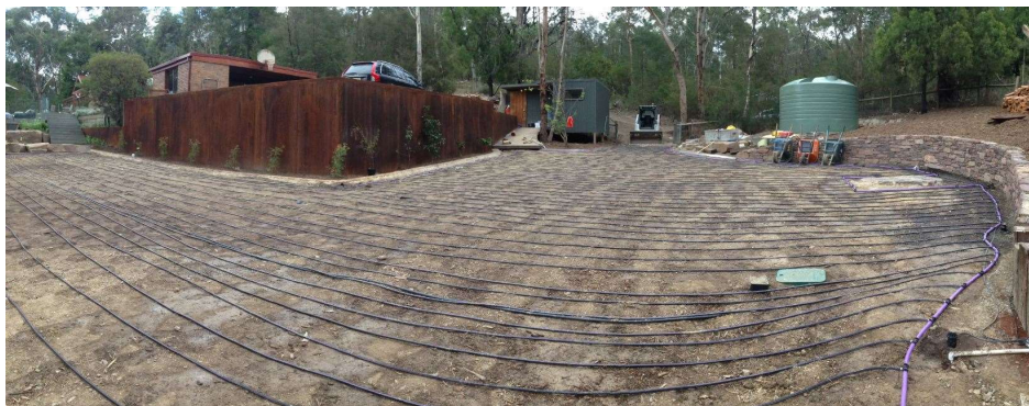
Figure 4: Lay-down of sub-surface irrigation
