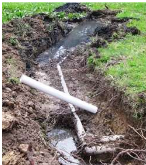
Figure 11: Flooded irrigation field and a deeply buried distribution pit (legacy system)
