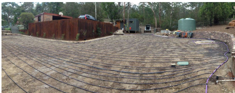
Figure 4: Lay-down of sub-surface irrigation
