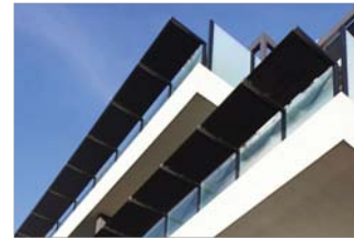
F10 1.2M HIGH OBSCURE GLASS BALUSTRADE WITH 0.6M DEEP HORIZONTAL LOUVRE SCREENING.
