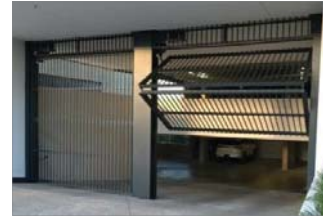
F09 SECTIONAL ROLLER DOOR WITH OPEN GRILLE PAINTED IN RESENE 'IRONSAND' N36-003-056.
