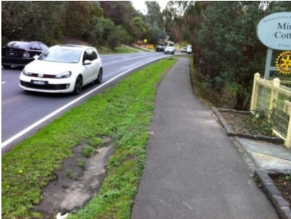
Roads with swale drainage systems
