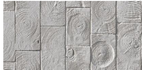
Concrete form texture example
