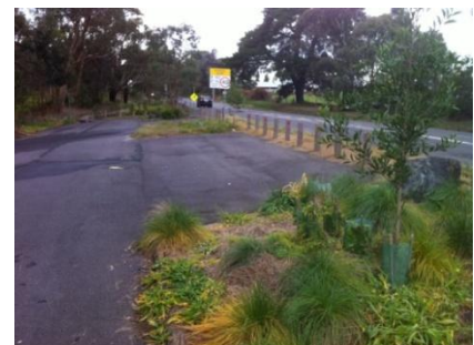
No car park line marking/kerb
