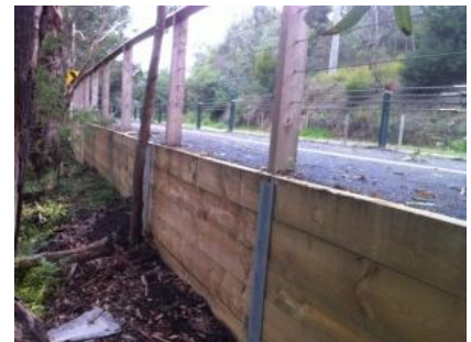
Simple timber sleeper walls
