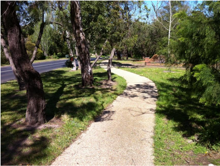
Exposed Aggregate Concrete High Use Footpath Example
