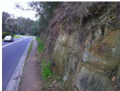
Exposed natural rock
