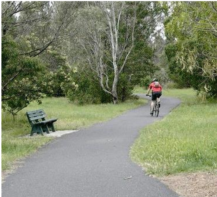
Asphalt High Use Shared Path Example
