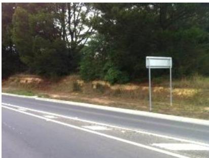
Stable natural roadside batters
