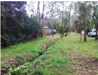
Open drainage networks
