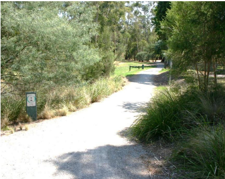
Aggregate Low Use Shared Path Example
