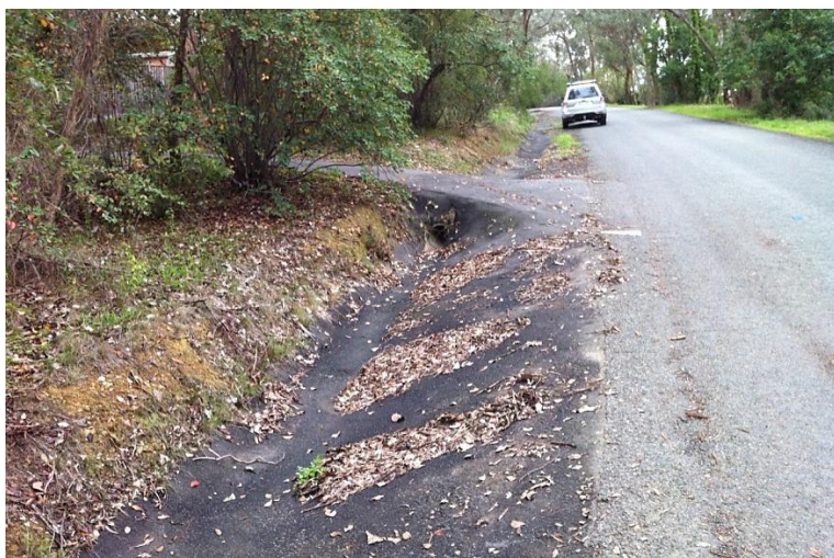
Asphalt Lined Swale Example
