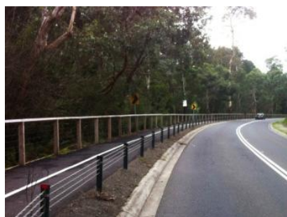
Wire rope barrier
