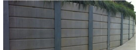
Concrete sleeper retaining wall
