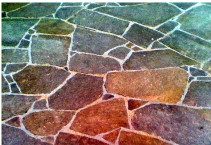
Traffic Management Pavement Examples
