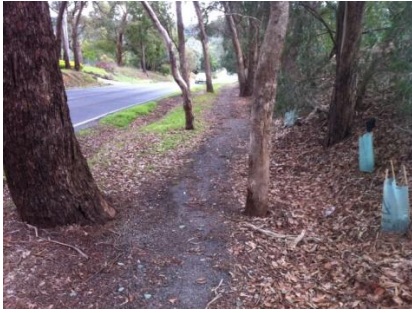
Aggregate footpaths in woodland street verge
