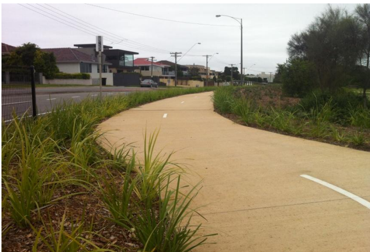
Coloured Concrete High Use Shared Path Example
