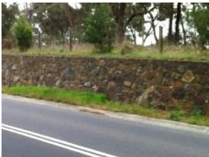
Rock-faced retaining walls in high visibility areas
