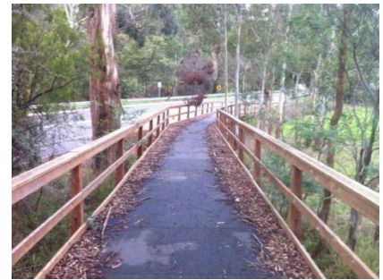
Boardwalks with composite deck and timber rails
