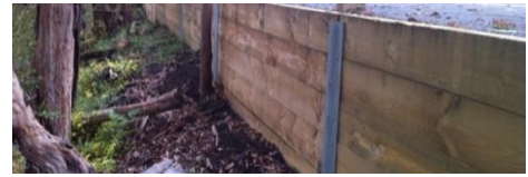
Timber sleeper retaining wall
