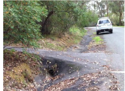
Culvert drive crossings
