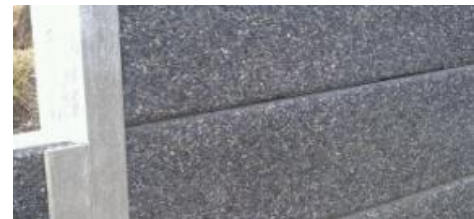
Concrete sleeper retaining wall
