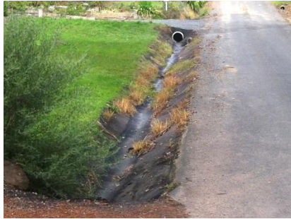
Lined table drains on steep streets
