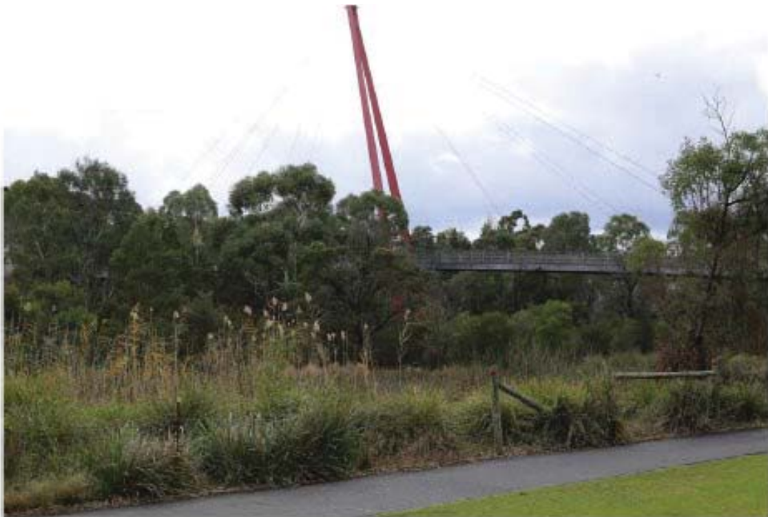
Figure 32: Technical Report H - Photo 9-33 'VP58 - Existing view north-east'
