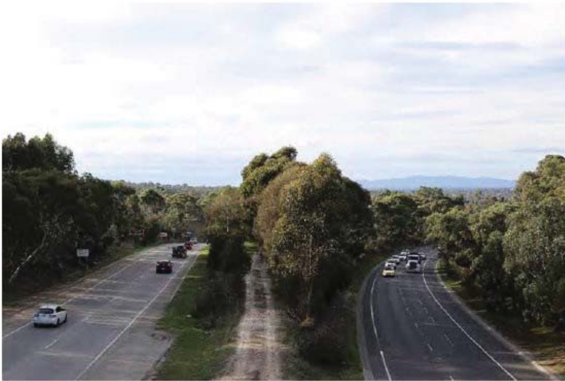
Figure 6: Technical Report H - Photo 9-47 'VP3 - Existing view looking south-east'
