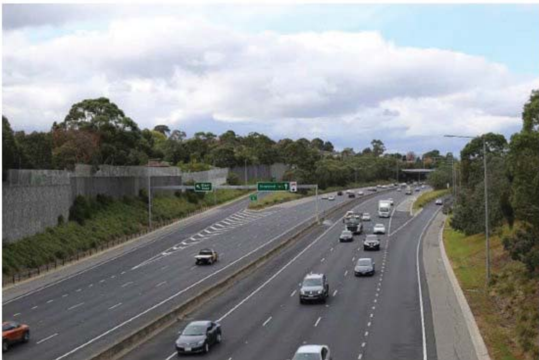
Figure 33 Technical Report H - Photo 9-34 'VP59 - Existing view looking east'
