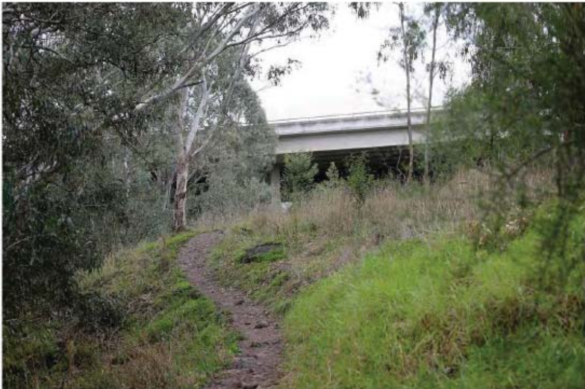
Figure 20: Technical Report H - Photo 9-21 'VP46 - Existing view south'
